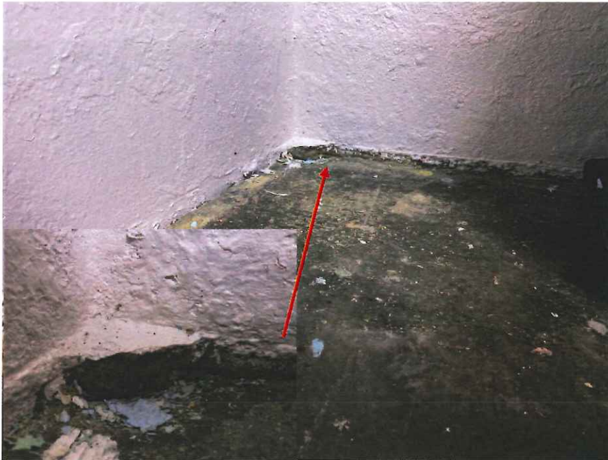
Photo 8: Undercut slab
